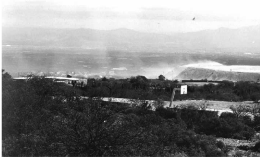
Figure 2. Aeolian dispersion of mineral particles from TD3 tailing pond towards the human settlement called Col. Real de Minas.
